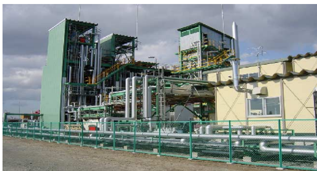
Fig. 1. Overview of JOGMEC GTL pilot plant (7 barrels per day).
